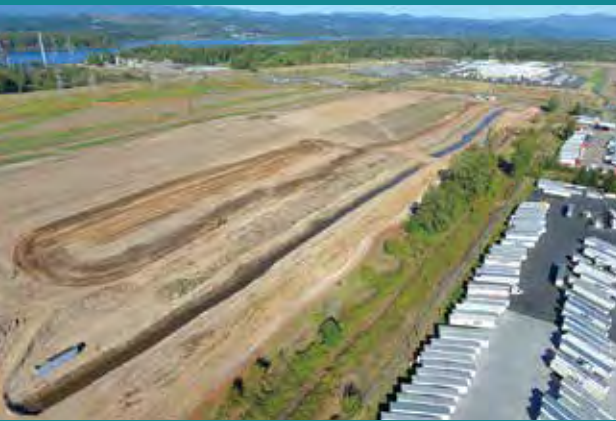
Troutdale Reynolds Industrial Park construction.
