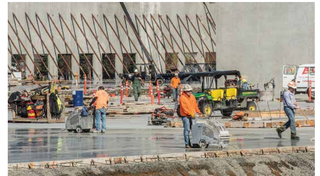
Subaru master parts distribution center takes shape at Gresham Vista Business Park.
