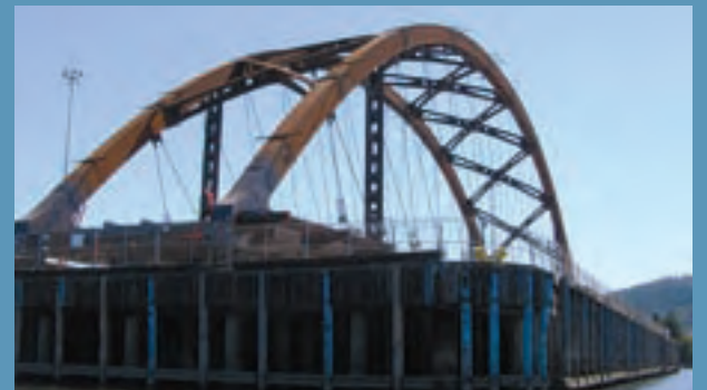
Bridge center span takes shape at T-2.
