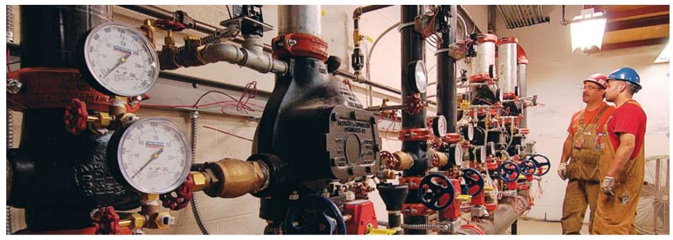
Workers complete the relocation of fire sprinkler piping prior to installation of a new in-line bag screening system at PDX.
