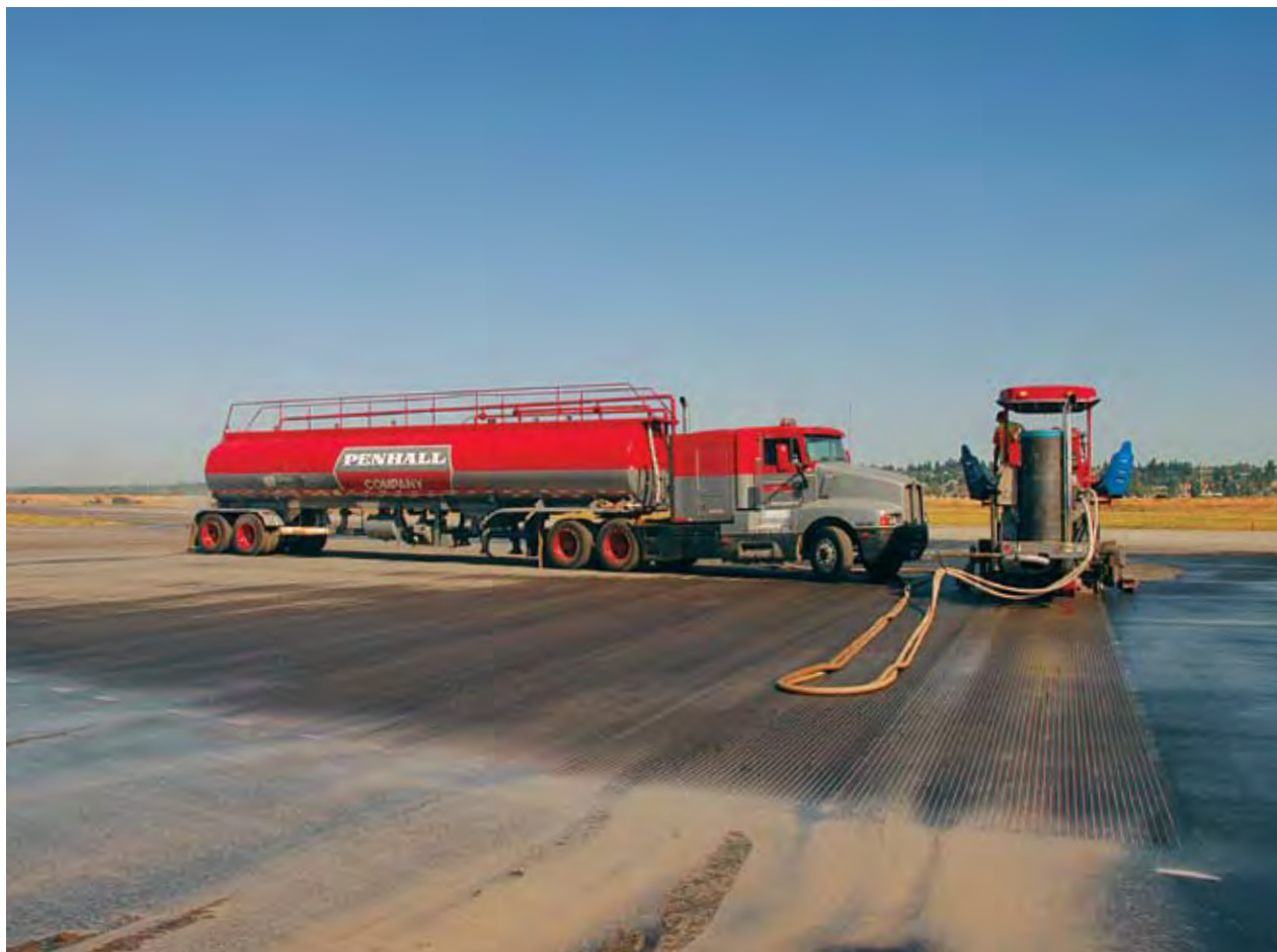
Equipment cuts grooves in newly-paved surface of north runway to facilitate rapid drainage of rainwater. Rehabilitation of the north runway is one of several capital projects under way at PDX.
