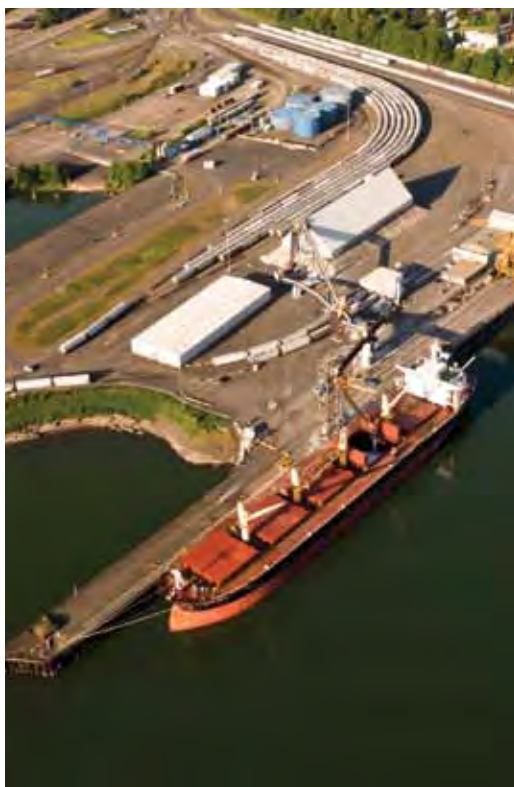
Terminal 4 soda ash export facility
