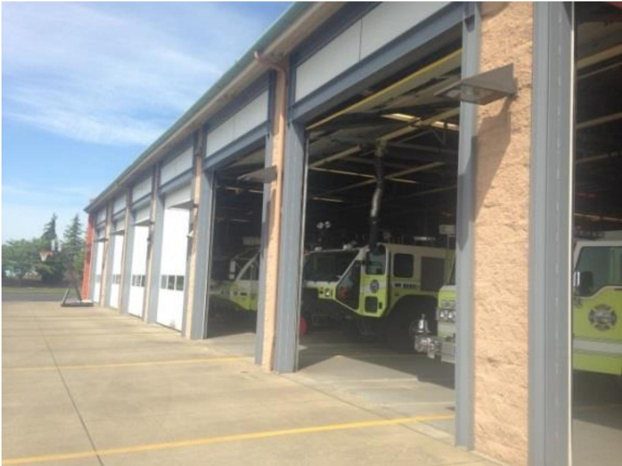
**Building Description:** The Fire Station is a single-story structure with two partial mezzanines and pitched roofs. The western portion houses the fire and rescue trucks.
