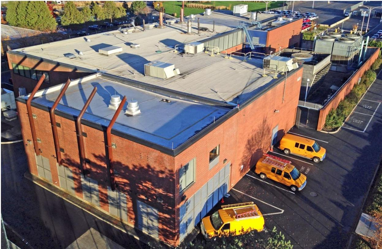
**Building Description:** The CUP is a one-story structure housing the airport’s central plant, including emergency utility systems, with a partial two-story office and storage section.
