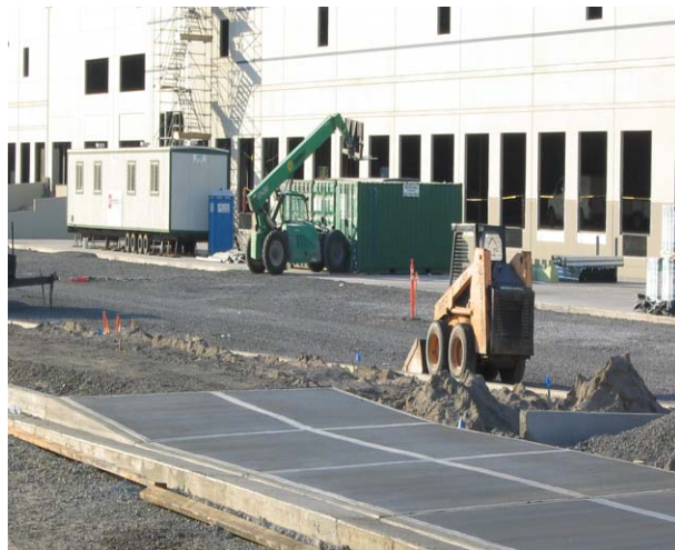
New construction in Rivergate.
