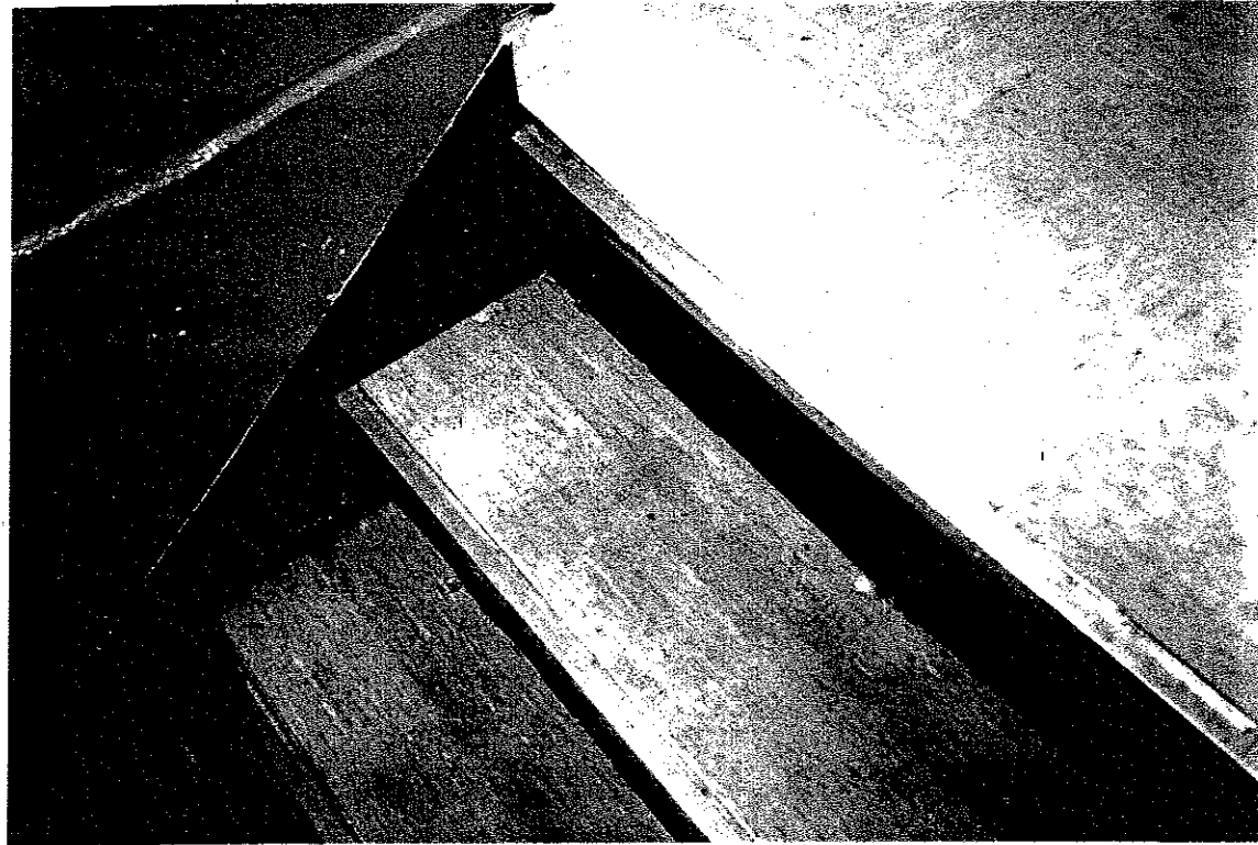
PHOTO 5: VINYL STAIR COVING; BLACK; LOCATED ALONG STAIRWELL WALLS IN WAREHOUSE 205 OFFICE; CONTAINS ASBESTOS; GOOD CONDITION.
