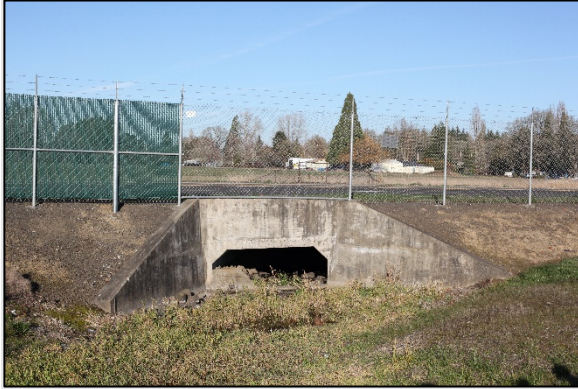
Looking north, Glencoe Swale passing under NE Evergreen Road
