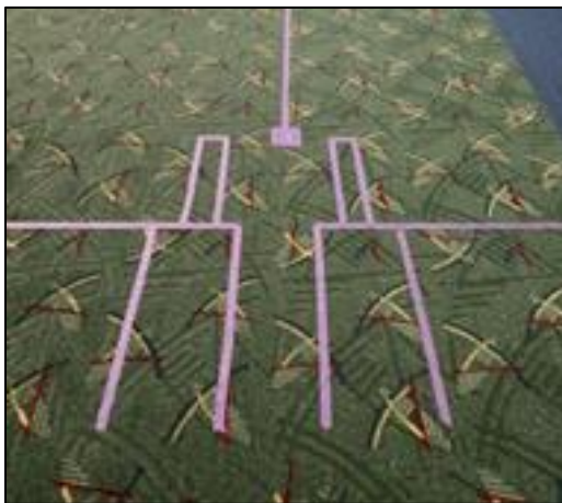
Survey markings in south tunnel in preparation for installation of new moving walkways.
