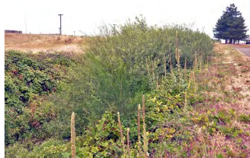
Figure A1-9. Drainage Ditch on ORANG Leasehold
