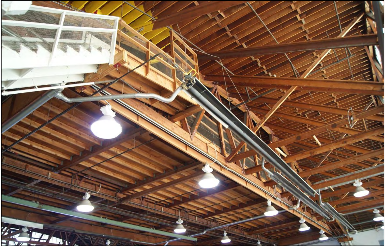
Figure 17. The timber framed loft that hangs from the roof trusses; the view is towards the east.
