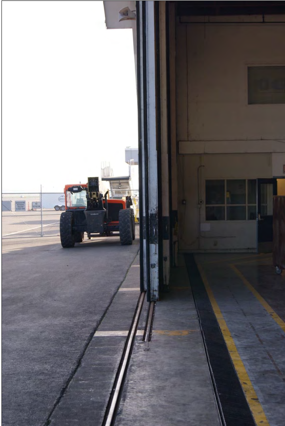
Figure 21. The sliding doors and the tracks set within the floor; the view is towards the east.
