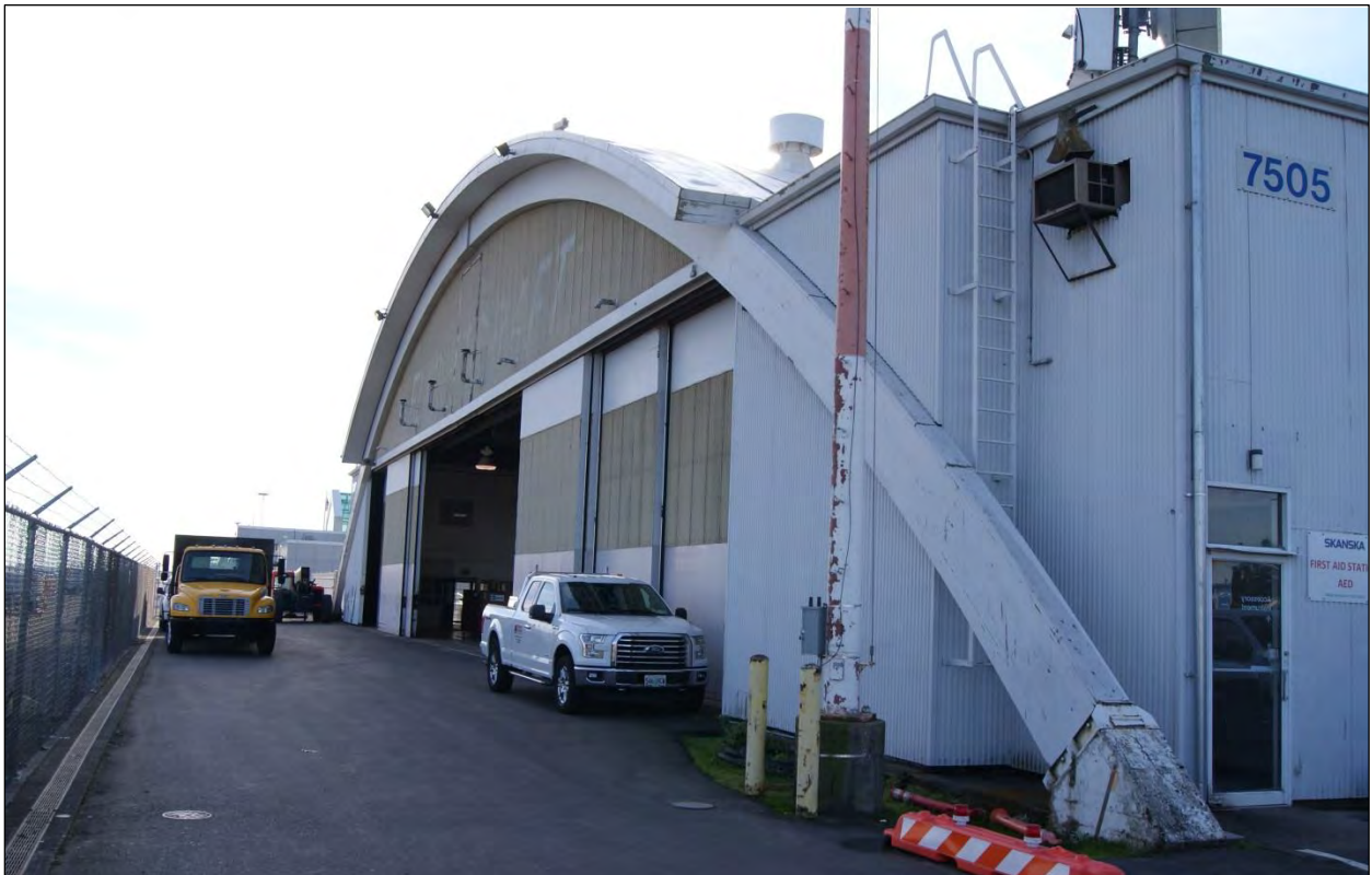
Figure 6. “A” Hangar’s north façade showing the exterior glulam arch; the view is towards the east.
