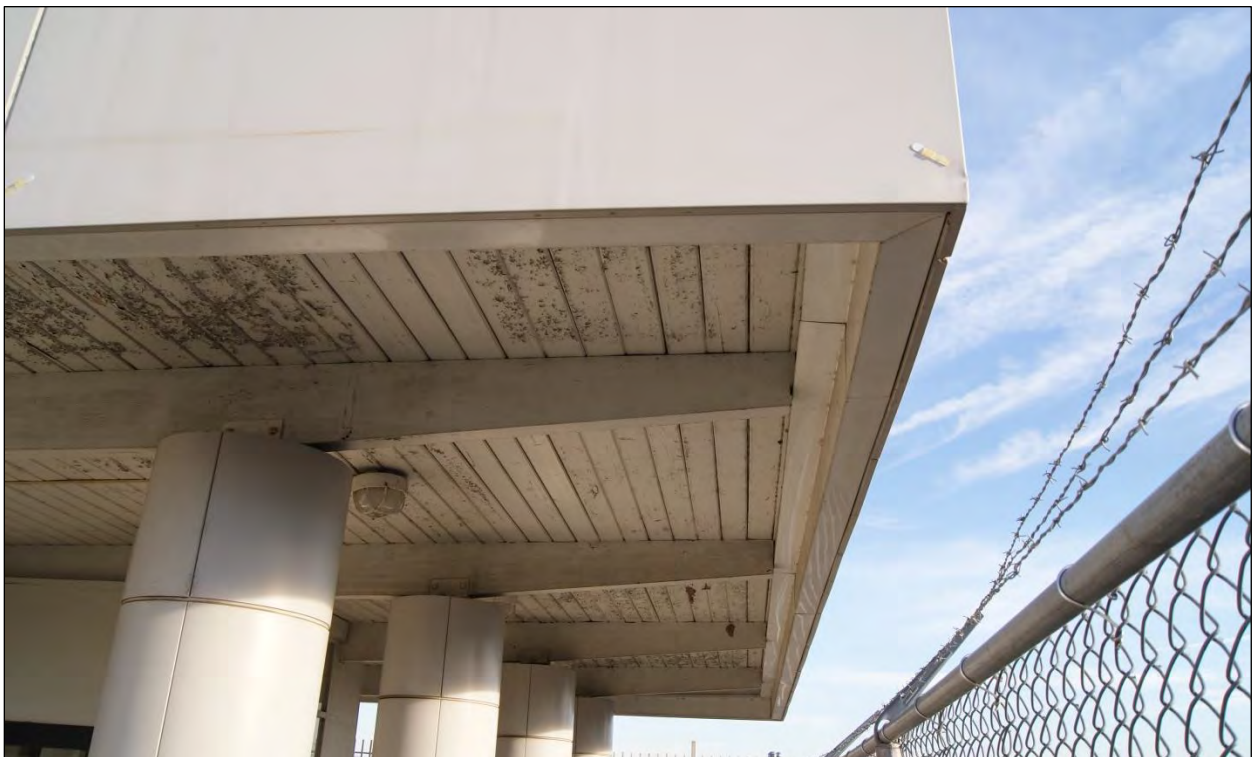
Figure 10. A detail of the entry canopy showing the original roof decking and supports; the view is towards the north.
