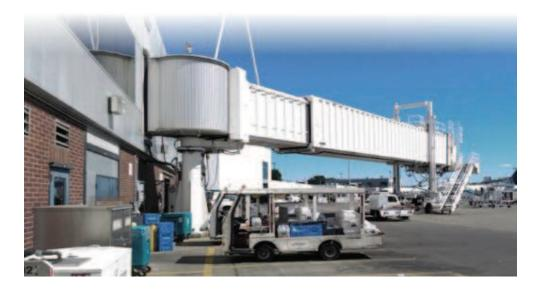
All but four of the PBBs at PDX were manufactured by JBT AeroTech. Mitsubishi, which no longer produces PBBs, manufactured the PBBs at Gates B1, B2, B3 and D2. The Gate B1, B2, and B3 PBBs were installed in 1986, and the Gate D2 PBB was installed in 1985. PBBs generally have a 30-year life expectancy.
