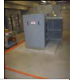
Parking Structure 1st Flr. SW Corner RM 1205B: P-1
